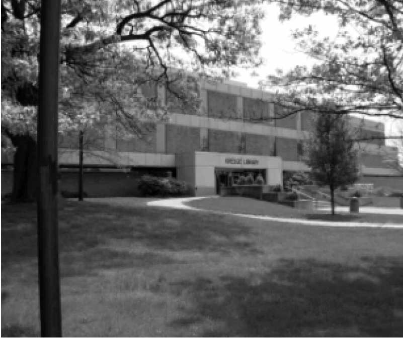
Figure 1. Kresge Library, originally built 1960–1962, greatly expanded 1987–1989 with the addition of the north and south wings. Photograph by Lisa Ngote.
